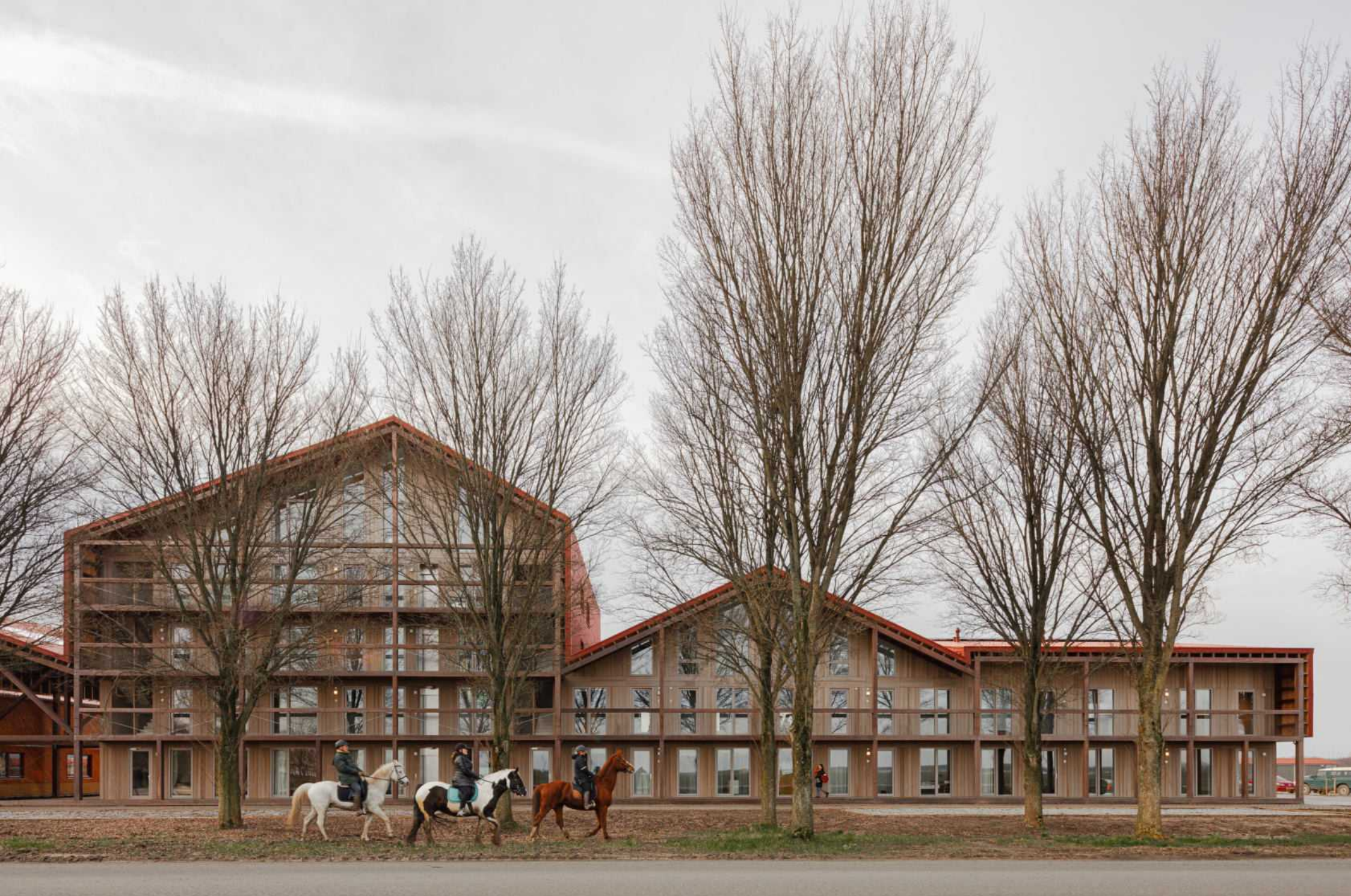
Vliervelden, Oosterwold, Almere, the Netherlands | A Gatehouse with 21 Apartments in a Farmyard | 2015 - 2022 | Client: Vink Bouw, Tom Saat and Tineke van den Berg
