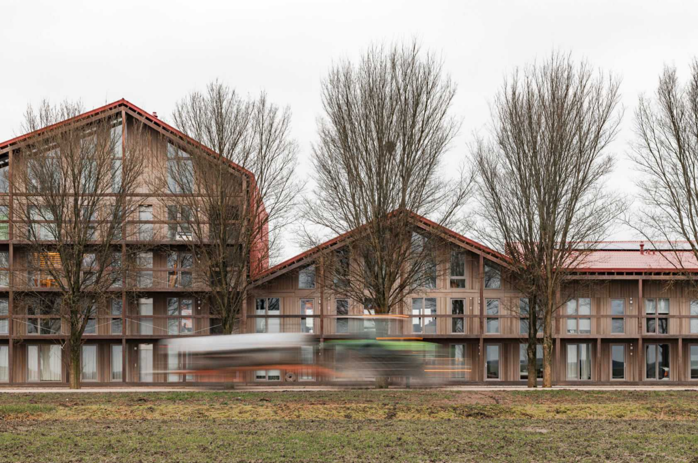
The galleries on the street side
