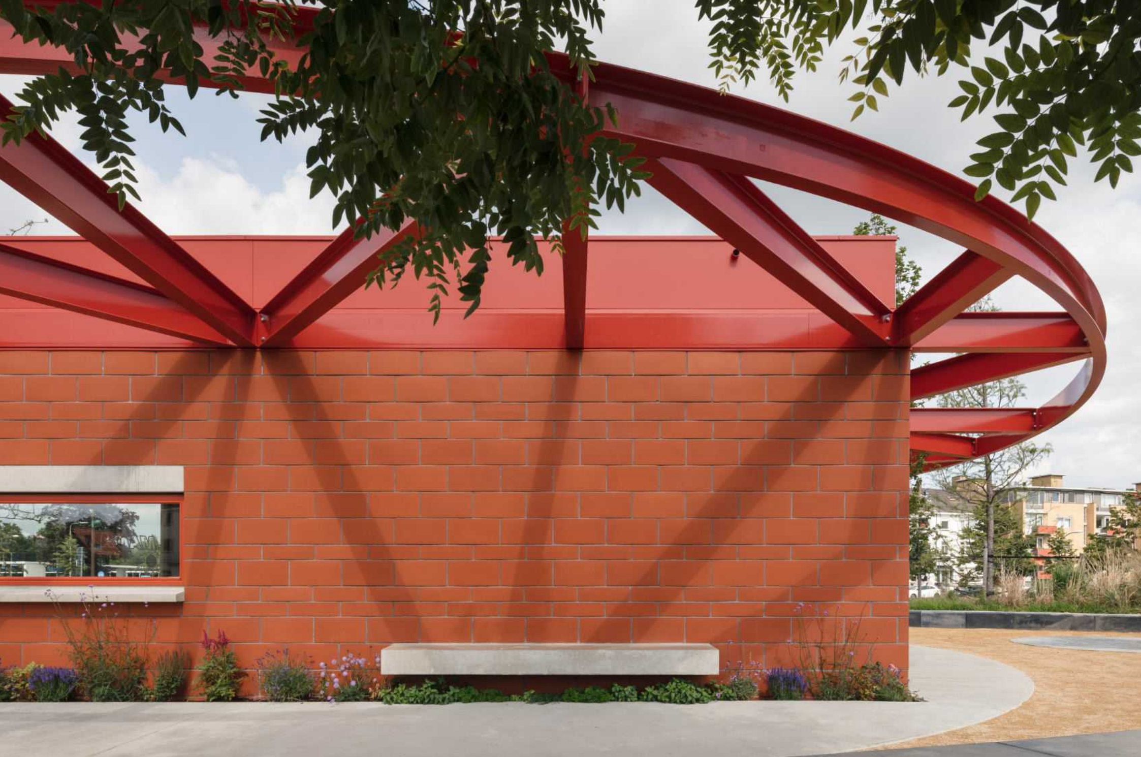
The brickwork façade is made with a leftover batch of terracotta module bricks from manufacturer Janinhoff. There were no fitting pieces or cornerstones available. Some of the blocks were therefore sawn, vertically or horizontally, to achieve the desired pattern, the dimensions of the façade and the position of the bench and window.
